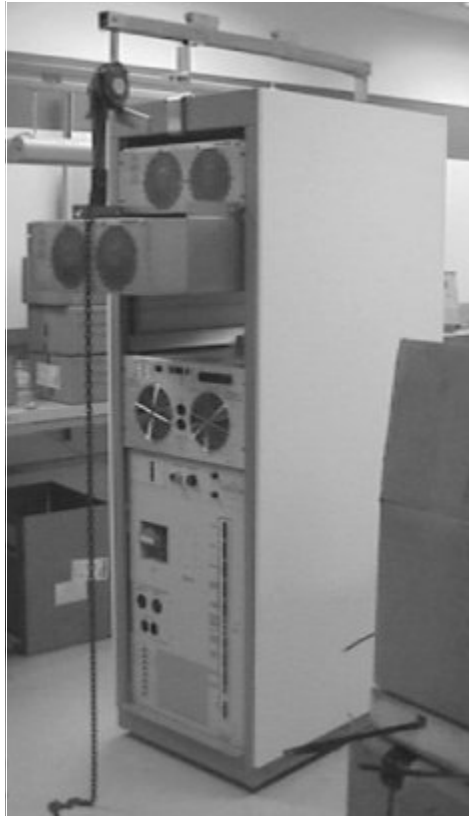
USING THE UNIVERSAL LIFT HOIST TO REMOVE THE RF AMP
