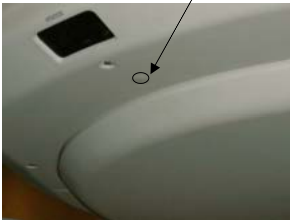
Old Ceiling Cover
