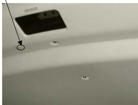
New Ceiling Cover
