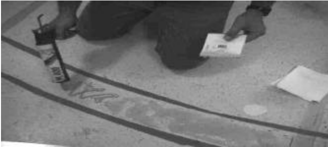
GLUING THE WEAR PLATE/RACE TO THE FLOOR ILLUSTRATION 1-13
