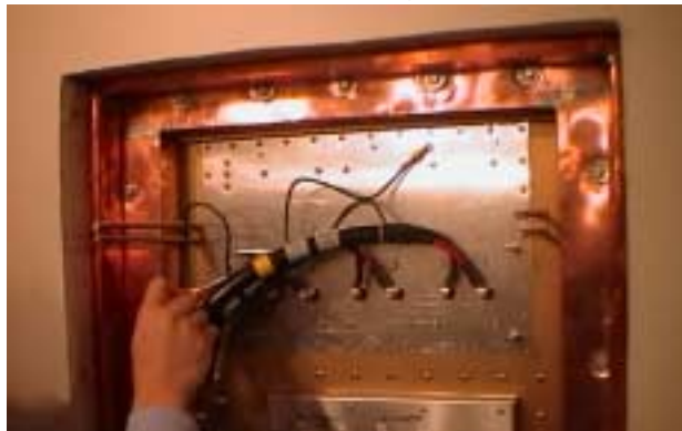
GRADIENT CABLE CONNECTION (SCAN ROOM SIDE) ILLUSTRATION 2
