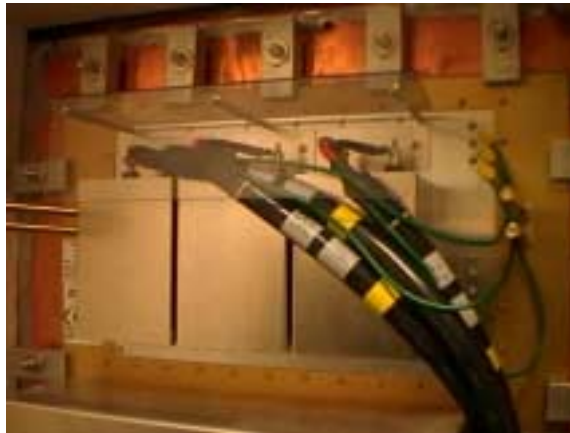
GRADIENT CABLE CONNECTION (MACHINE ROOM SIDE) ILLUSTRATION 1
