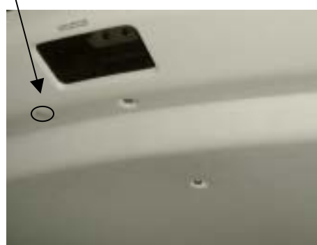
New Ceiling Cover
