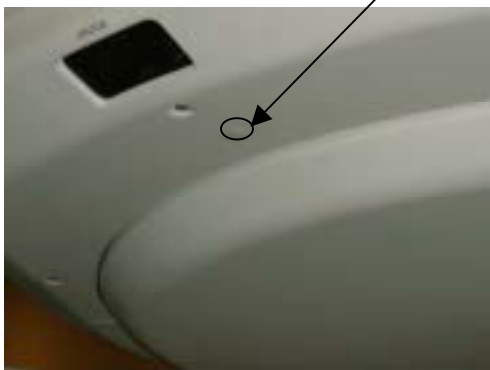
Old Ceiling Cover
