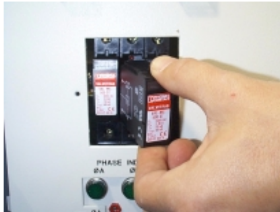
TVSS MODULE REPLACEMENT ILLUSTRATION 4–2
