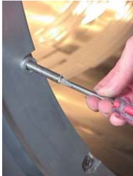
TIGHTENING STUD ILLUSTRATION 3-8
