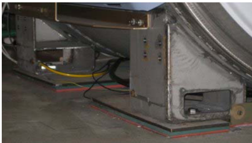
Figure 6-9 Magnet installed on surface mounted non-SV vibroacoustic damping mats
