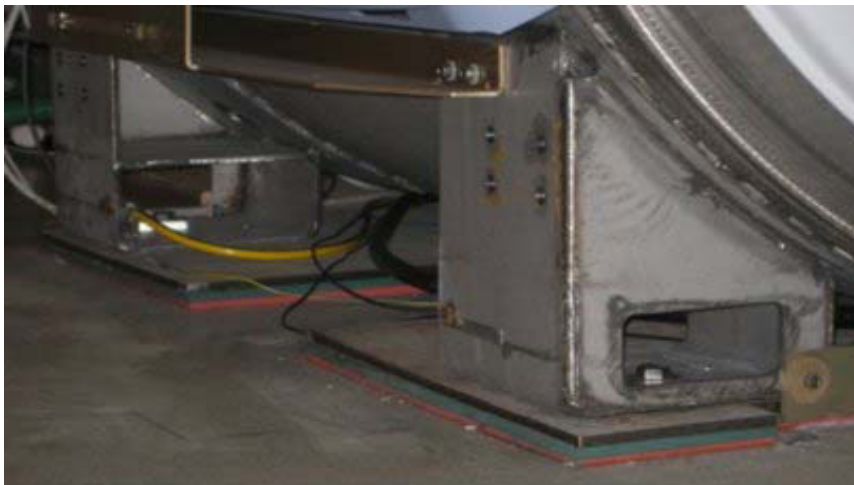
Figure 7-11 Magnet installed on surface mounted non-SV vibroacoustic damping mats
