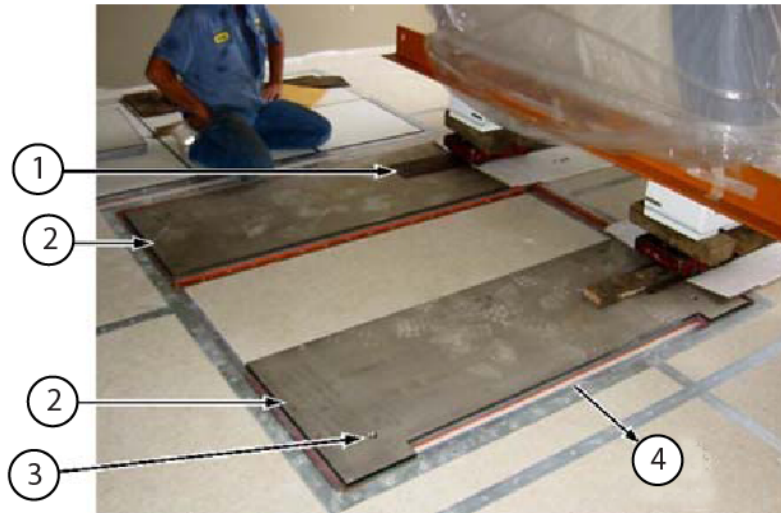
Figure 7-10 Moving the magnet onto surface mounted non-SV vibroacoustic damping mats
