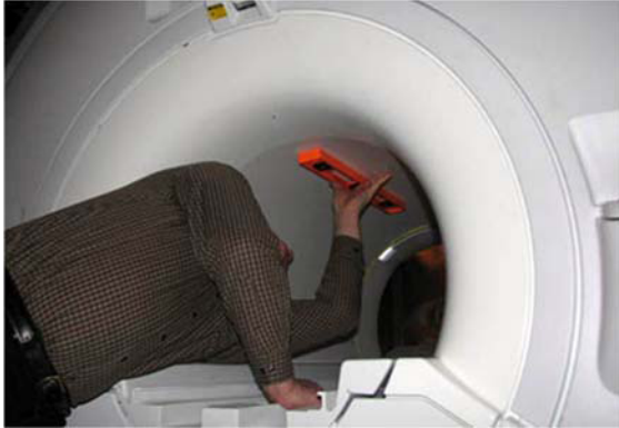
Figure 6-12 Magnet leveling, front-to-back
