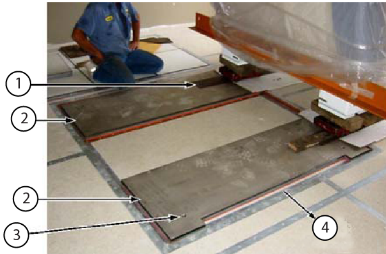
Figure 6-8 Moving the magnet onto surface mounted non-SV vibroacoustic damping mats
