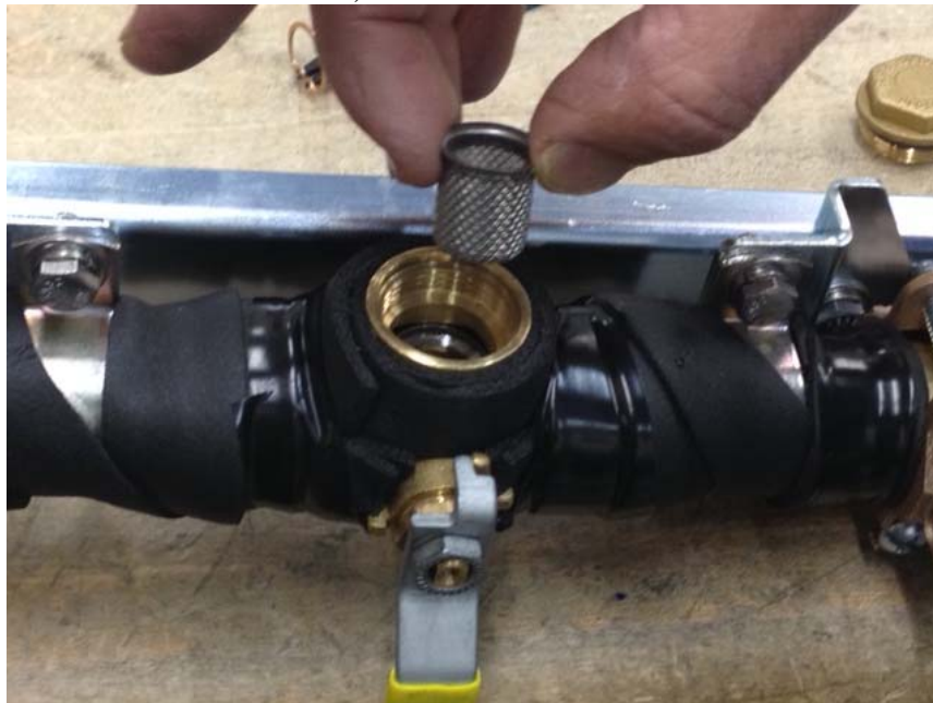
Illustration 6: Configuration #2 Removing Strainer Basket from Valve
