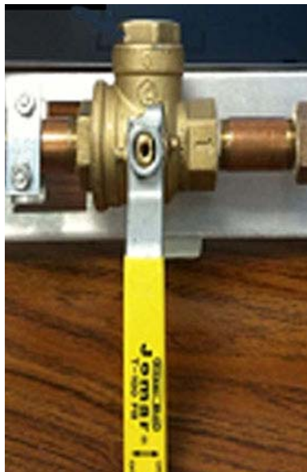
Illustration 4: Configuration #2 Filter Ball Valve Closed
