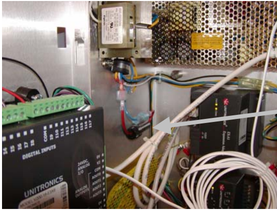
Photo 3 Older Style In-line Fuse holder.
