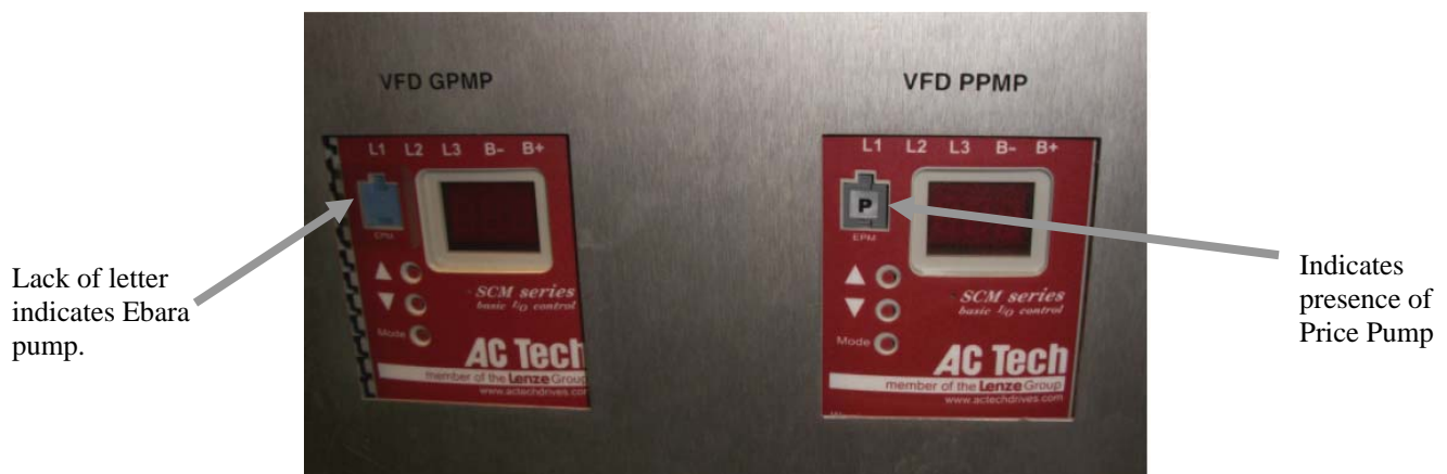
Photo 1 Detail of VFD EPM Chip in different Pump Style VFDs
