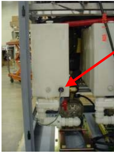
Illustration 2 DI Sensor Location
