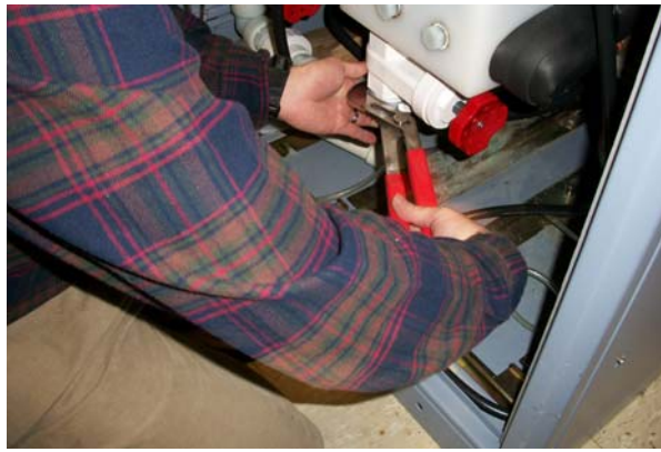
Figure 2 Installing new hose bard fitting detail.
