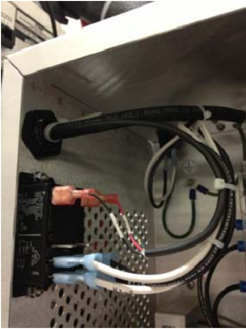
Photo 5 Close-Up of J1 zip ties in power box
