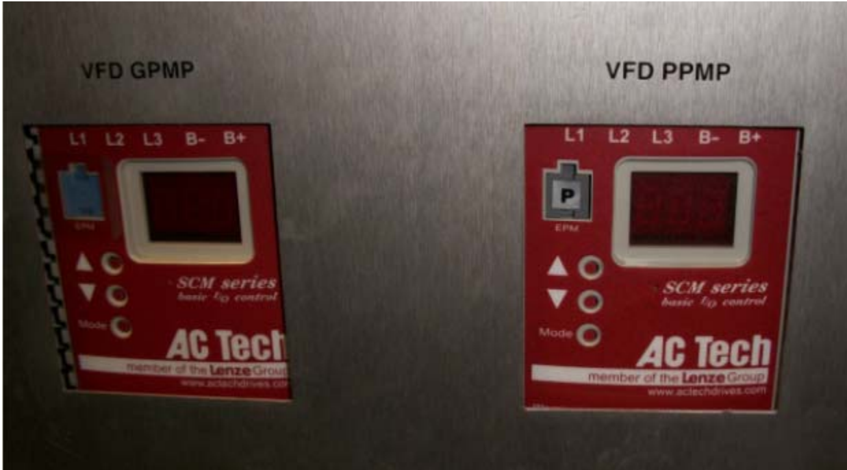
Figure 7 Complete installation. (This HEC has an Ebara gradient coil pump and a Price power electronics pump, as noted by the 'P' on the VFD chip in the power electronics VFD)
