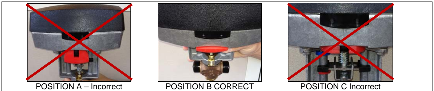
Illustration 8 – Manual/Auto Switch Position on Mixing Valve
