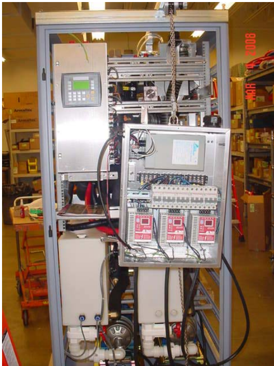
Photo 5 Lowering Power Box to floor
