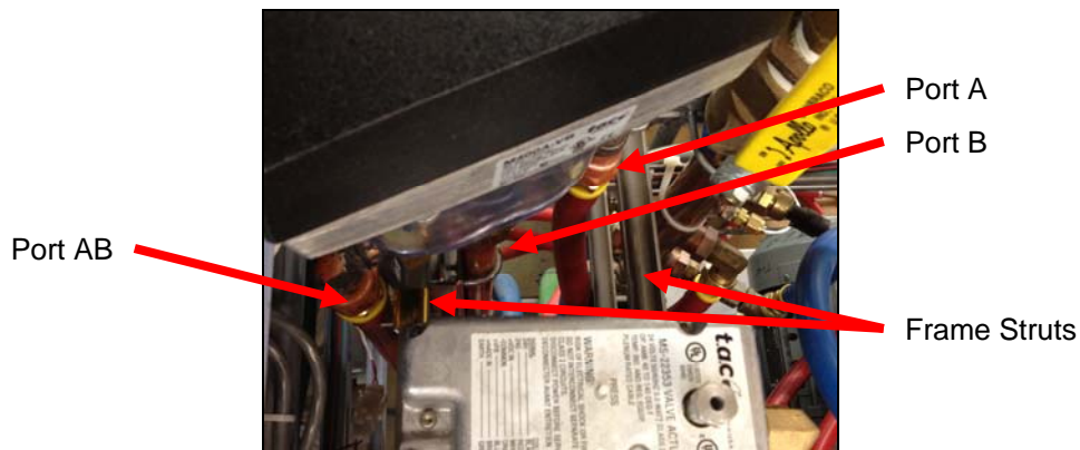
Illustration 8 – New Style Valve Installed in G6000EN Cabinet (System without Insulation)
