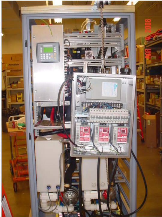
Figure 5 Lowering Electrical Box to floor.
