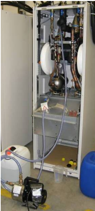
Figure 19 - GC filling setup
