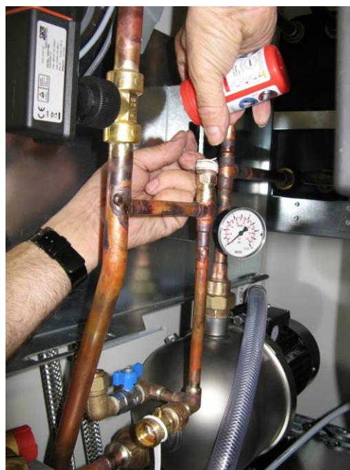
Figure 70 - Wind with Loctite 55
