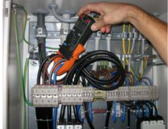
Figure 6 – HIOKI clamp-on leak tester for gMDU
