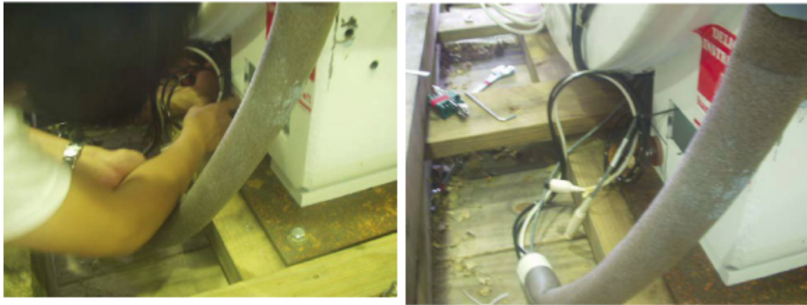
Illustration 2-80: Withdrawing PAC Interface Cables
