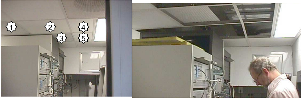
CEILING TILES REMOVED ILLUSTRATION 1-4
