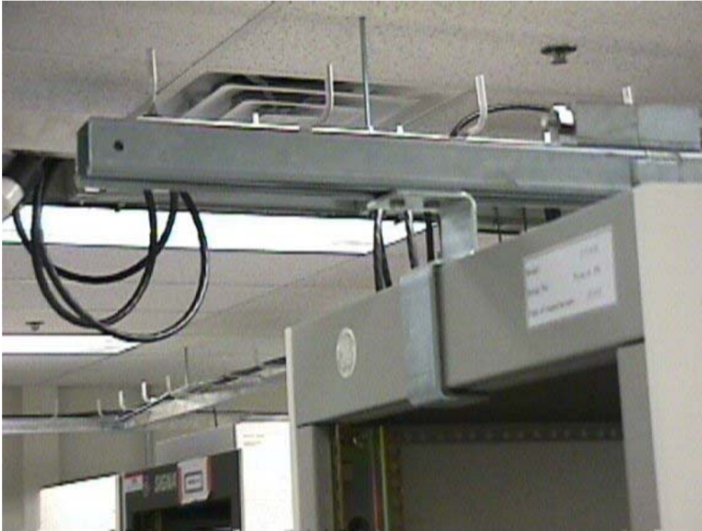
HOIST INSTALLED ON ACGD LITE CABINET ILLUSTRATION 1-7
