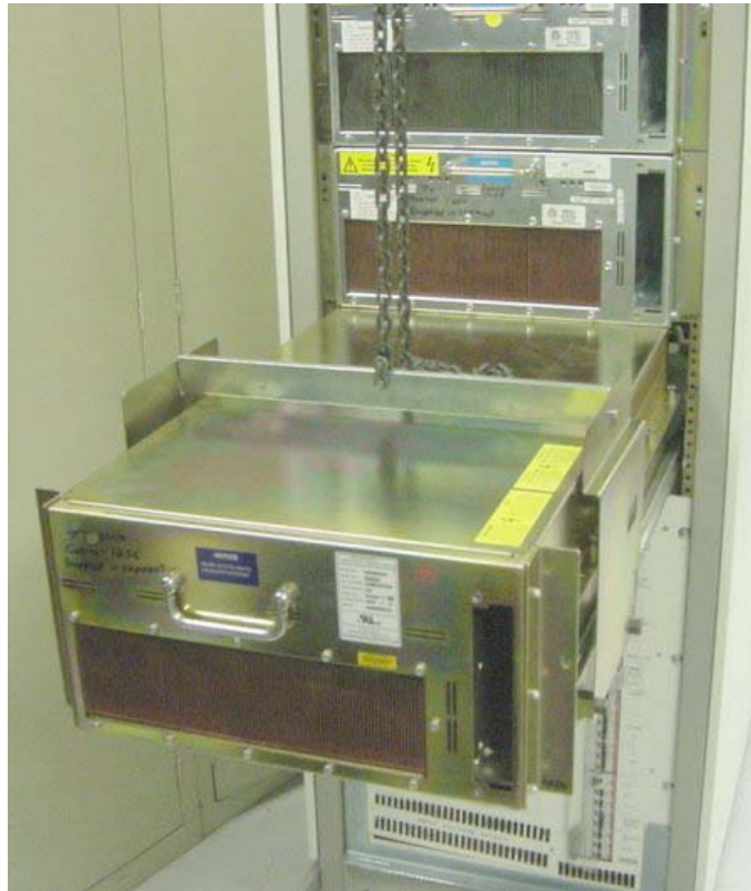
ATTACHING THE SPREADER BAR TO THE HOIST BRACKETS ILLUSTRATION 1-19
