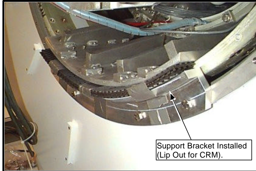
SUPPORT BRACKET INSTALLED
