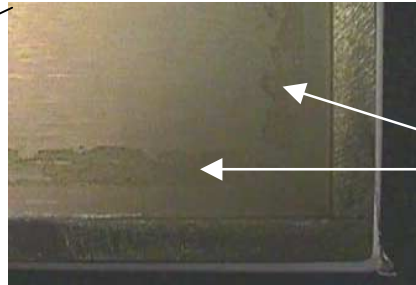
REMOVE OLD GLUE RESIDUE ILLUSTRATION 1-2
