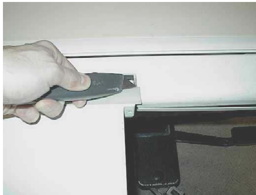
CUTTING BUMPER ENDS
