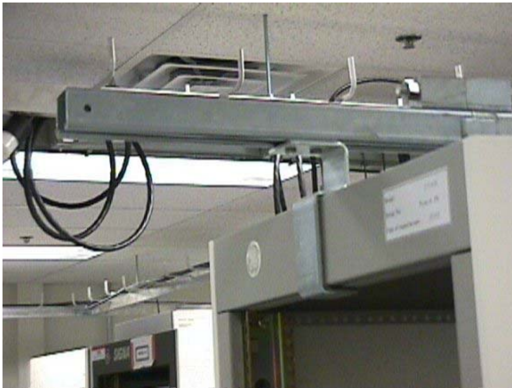
HOIST INSTALLED ON ACGD LITE CABINET ILLUSTRATION 1-5
