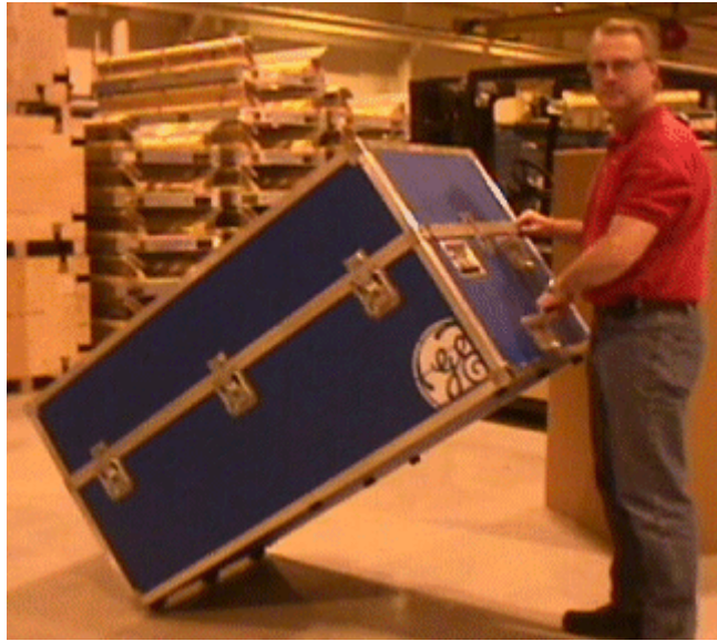
MOVE RF COIL CASE TO FINAL LOCATION: SET CASE HORIZONTAL ILLUSTRATION 4-2
